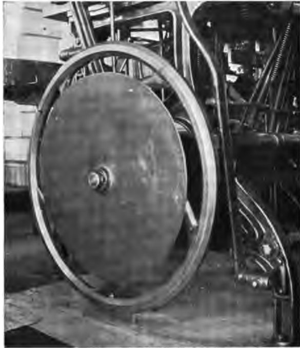
Fig. 4. Fly-Wheel Guard.
